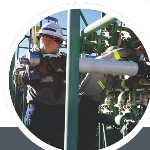
Membrane change out and installation of Xebec hollow fibre polyimide membrane
